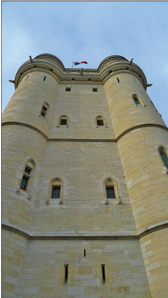
The donjon tower of the Château de Vincennes, in Paris, is 52 meters high and represents the tallest medieval fortified structure in Europe. King Philip VI of France started this work about 1337. The work was completed during Charles V's reign. When Nicole Oresme was a scholar in Paris, this donjon was in the process of being erected. Later on, during the reign of Charles V, this donjon served as a residence for the royal family. Its buildings are known to have once held the library and personal study of Charles V.
