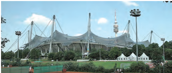
Figure 4. Frei Otto modeled the Olympic stadium in Munich on minimal surfaces.
